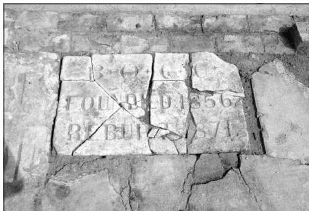
Corner stone of the BME, unearthed in its cellar. Photo: Infrastructure Ontario
